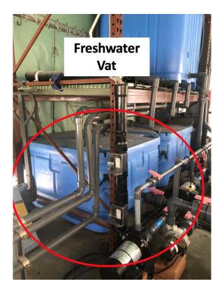
6) Turn these valves vertically, so they start pumping freshwater into the freshwater vat. Wait until the vat is completely full.
