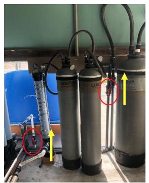
7) Make sure all these valves are open. If one of these is not open, it could cause the pump to run dry.
