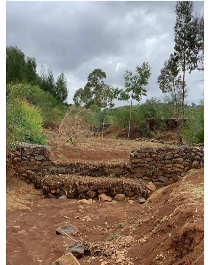
Gabion check-dam
